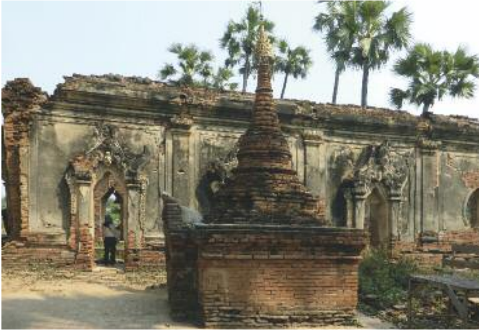
Fig. 10.16 Yadana Hsemee Pagoda Complex, Innwa, with extensive losses of plaster cladding.
