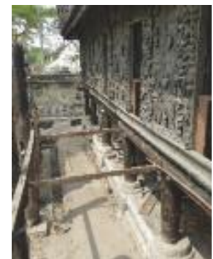
Fig. 10.11 Replacement of the base of pillars with concrete, Shwenandaw Kyaung, Mandalay.
