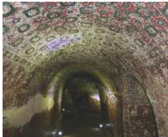
Fig. 10.17 Me Nu Ok Kyaung Innwa, signs of leakage in the vault of interior hallway.
